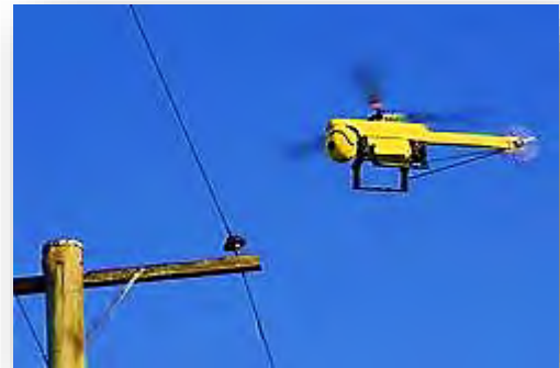
Increasingly, UAVs or Drones are being used to inspect powerlines. Avista plans to deploy this technology as part of Wildfire Resiliency.
